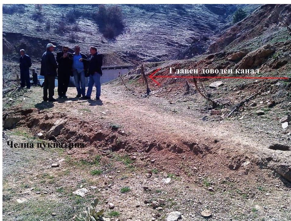
Figure 20. Current state of the landslide (source: photographed 29.03.2012)
