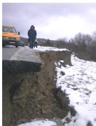
Figure 8. Secondary landslide fracture on 21.02.2010
