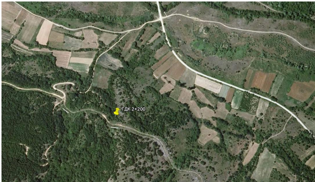
Figure 12. Landslide location (source: Google Earth)
