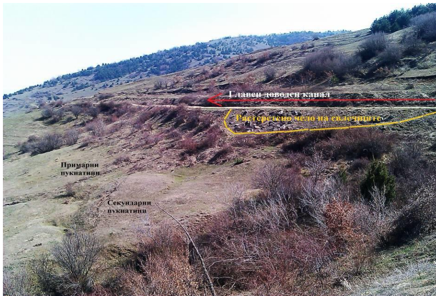
Figure 17. Current state of the landslide (photo 29.03.2012)
